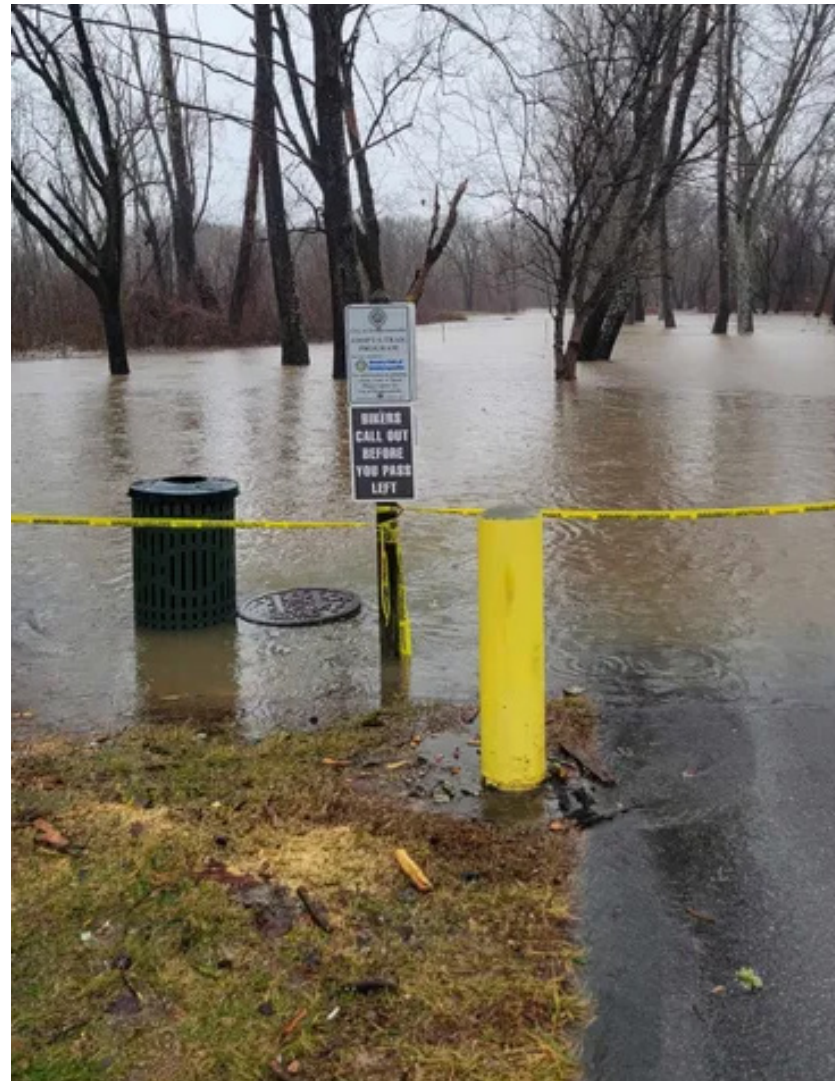
Image 47. Flooding on the Oklawaha Greenway (2024)
