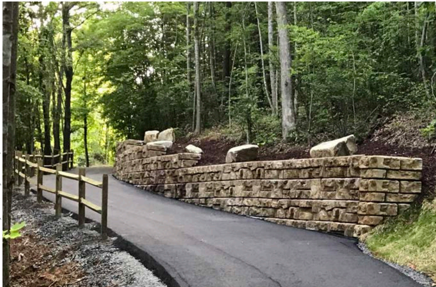
Image 46. Retaining Wall Example (Purple Martin Trail)
