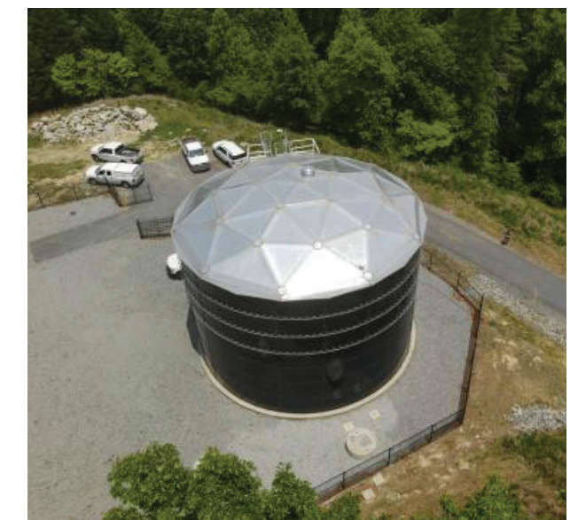
Water storage tank | City of Hendersonville
