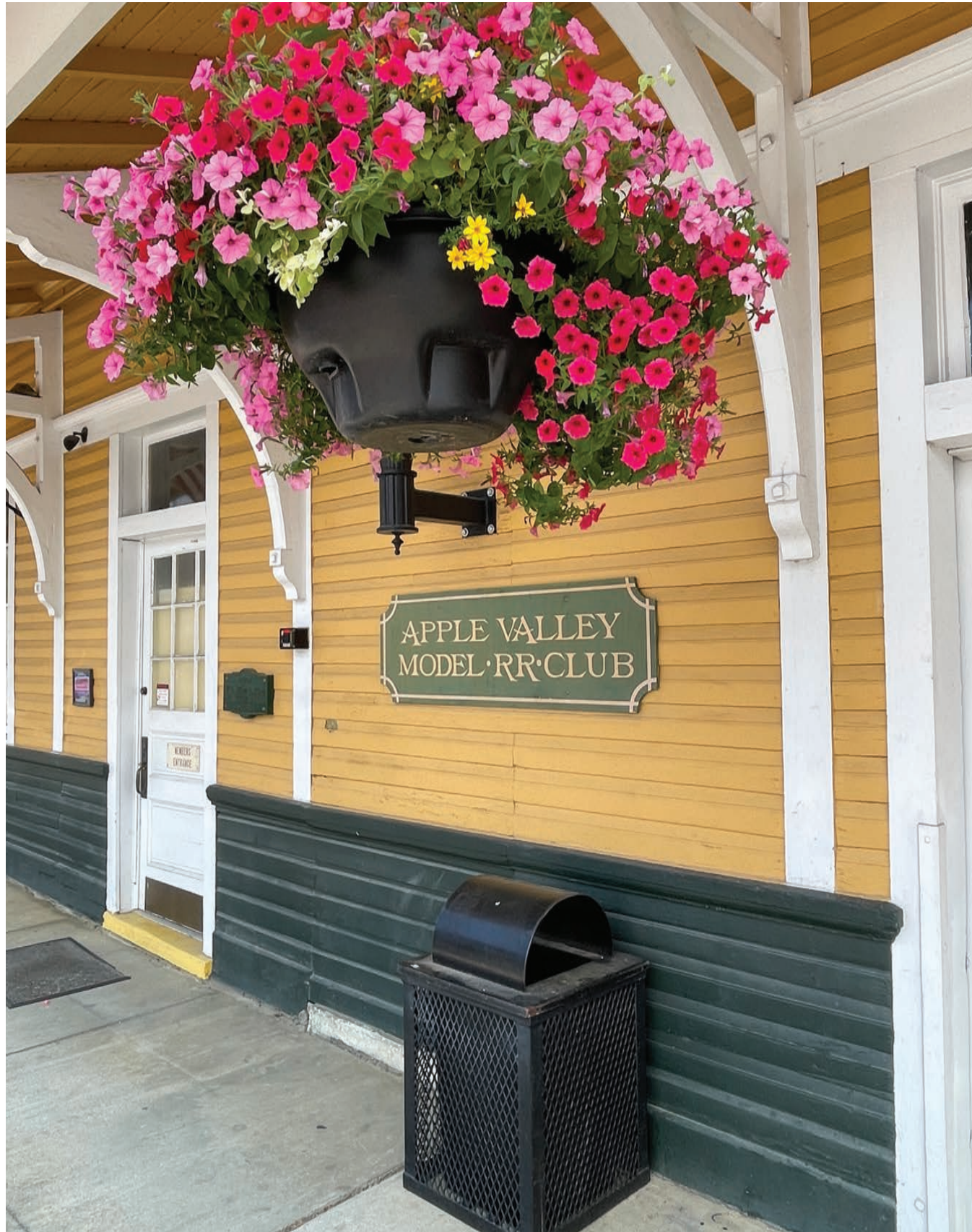
Historic Depot building
