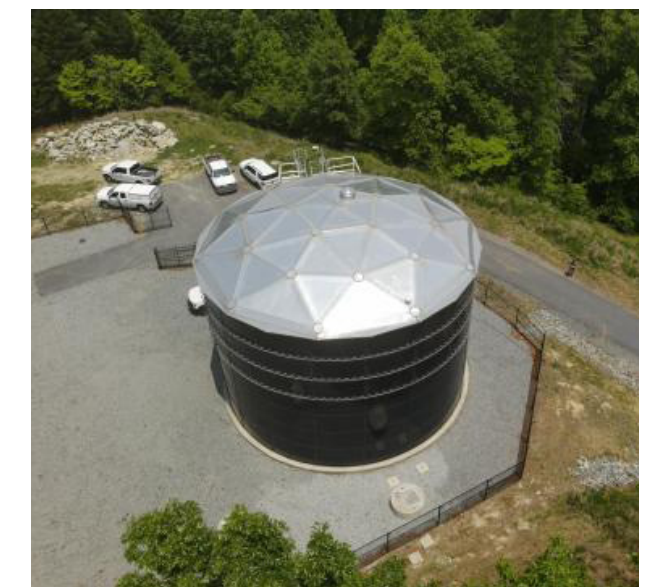
Water storage tank | City of Hendersonville
