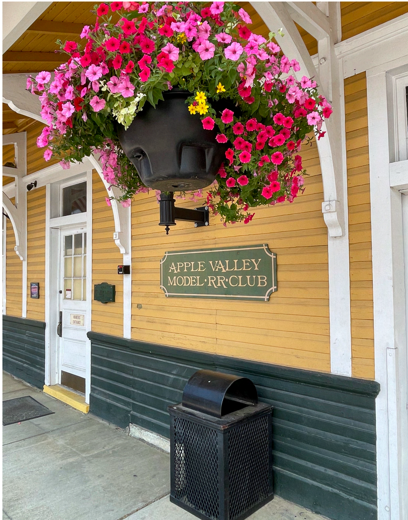
Historic Depot building
