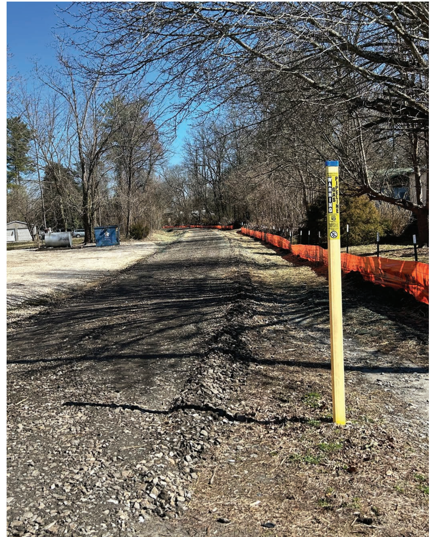
The Ecusta Trail under construction
