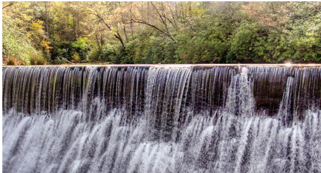
Hendersonville water supply | City of Hendersonville
