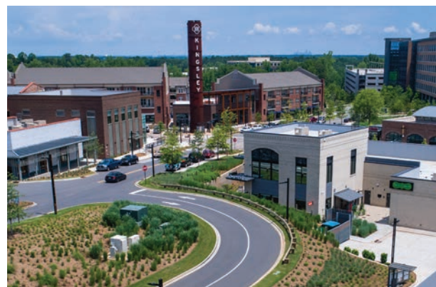
Kingsley Mill | Kingsley Fort Mill, SC
