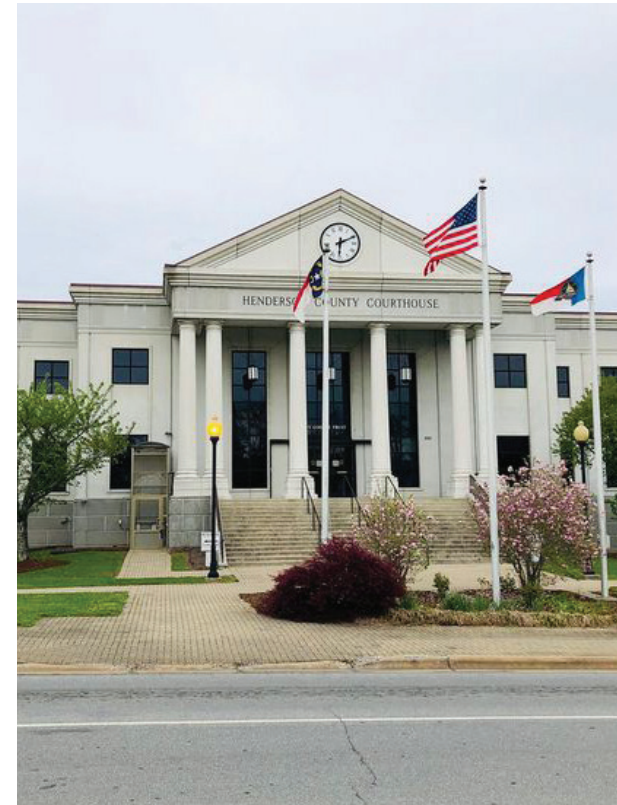
Henderson County Courthouse | Flickr, Devtmefl
