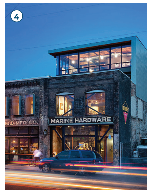
New infill or additions can be sensitive to the existing character. Kolstrand Building | Aaron Lietz
