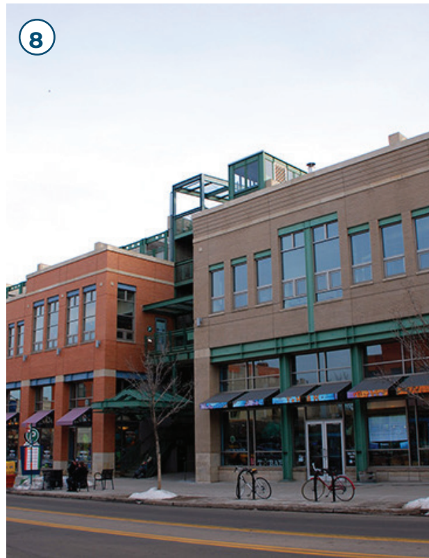
8 Shared parking can be integrated into other uses such as retail or housing. 15th and Pearl Parking Deck in Bolder | Build Better Burbs
