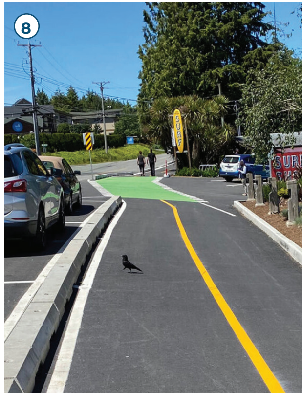
8 Streetscape improvements change the aesthetic along major arterials | Hazelwood Construction Services
