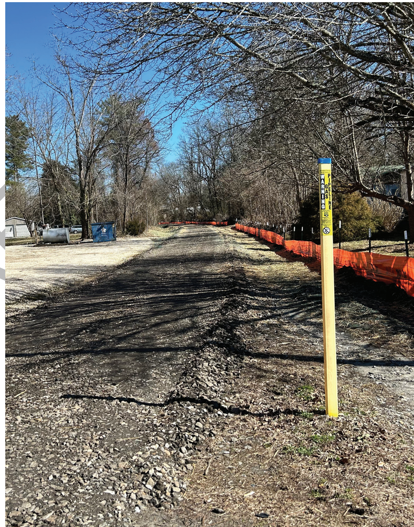
The Ecusta Trail under construction
