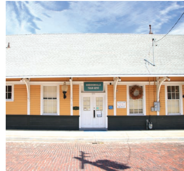
Hendersonville Train Depot | Visit Hendersonville
