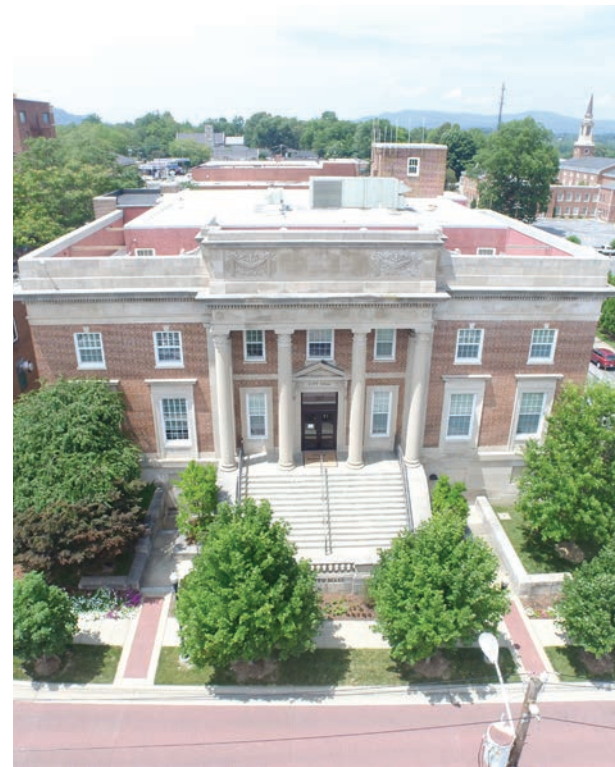
Hendersonville City Hall | City of Hendersonville
