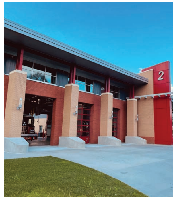
Fire station | City of Hendersonville
