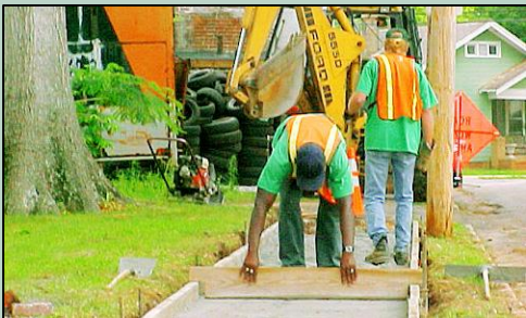
Example of sidewalk construction
