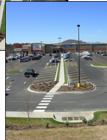
Example of pedestrian channels in parking lots
