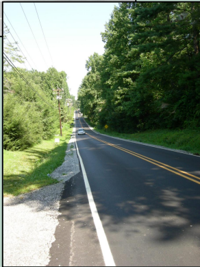
Lack of sidewalks on Haywood Road and Blythe Street
