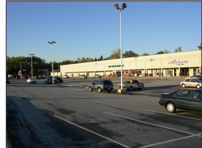
Safe pedestrian access is limited in this shopping center
