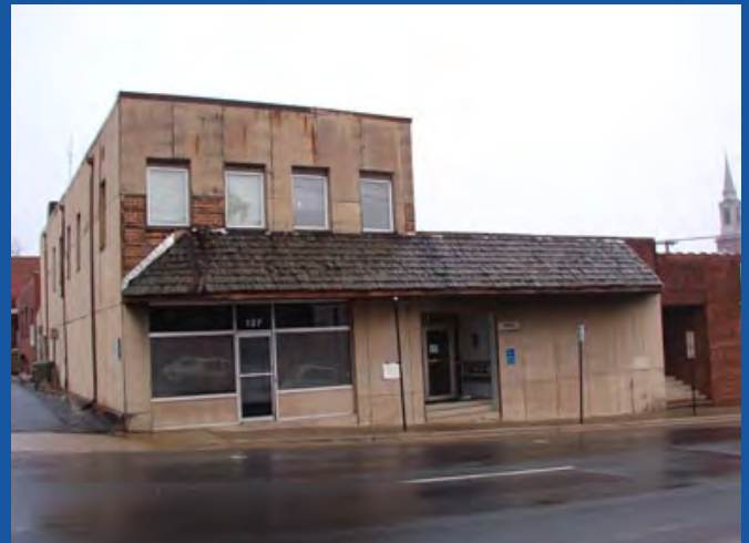
Former Times News Building, Housed PD from the late 1960s - 2005
